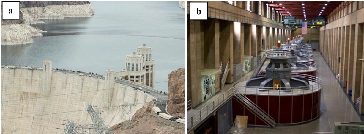
Figure 5.11. a) A view of the Hoover dam from above (credit Adam Kliczek). b) Hydroelectric generators at the Hoover dam (credit: Jon Sullivan).
