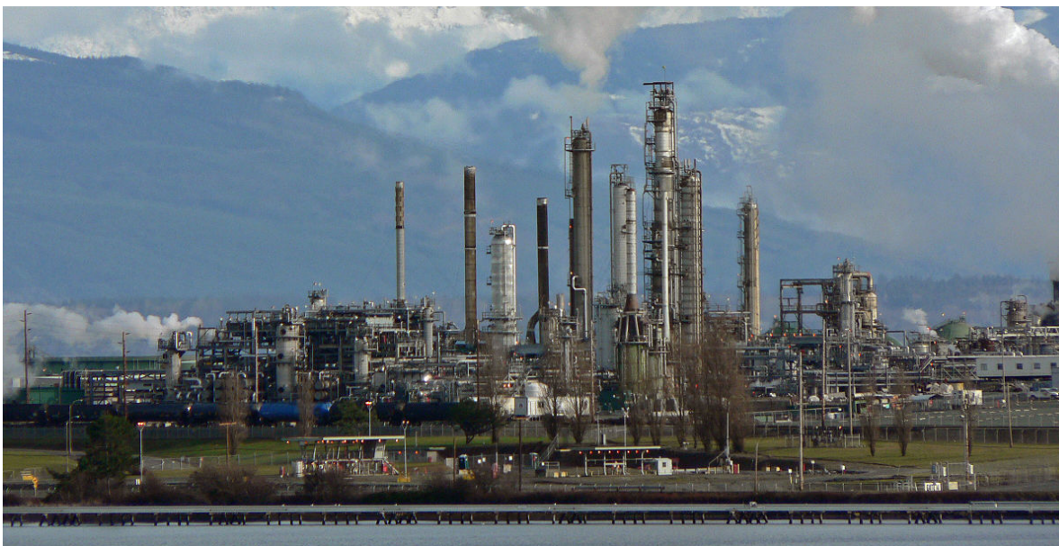
Figure 4.8: Tesoro Corporation Oil Refinery in Anacortes, Washington. Photo by Walter Siegmund. https://commons.wikimedia.org/wiki/Oil_refinery#/media/File:Anacortes_Refinery_31904.JPG
