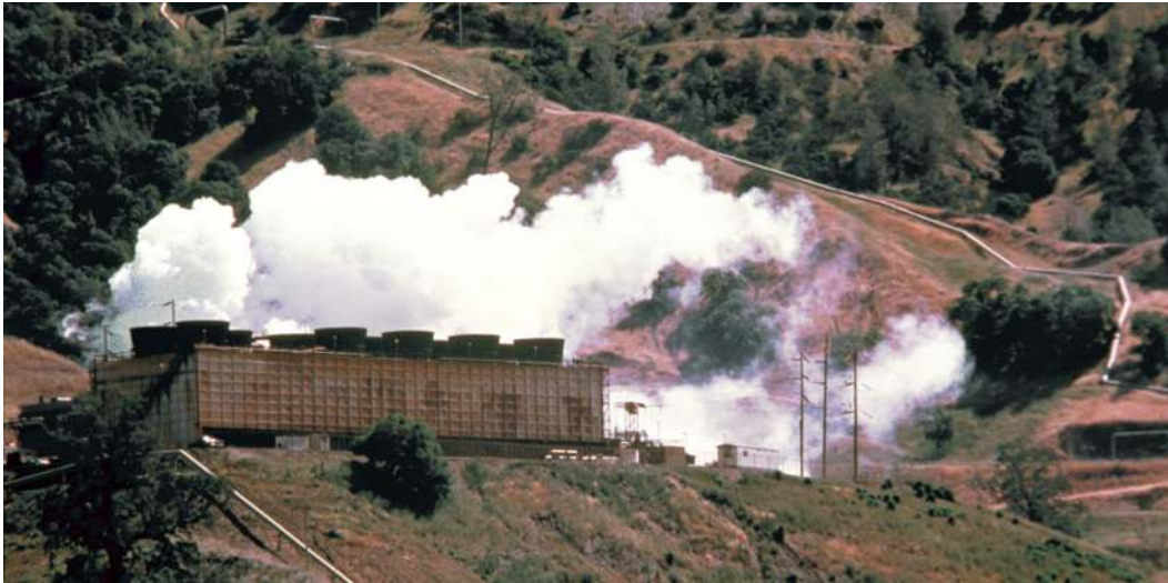
Figure 7.1 This geothermal energy plant transforms thermal energy from deep in the ground into electrical energy, which can be easily used. (credit: modification of work by the U.S. Department of Defense)
