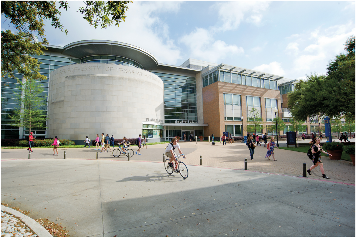
Chemistry-Physics Building with the new Planetarium
