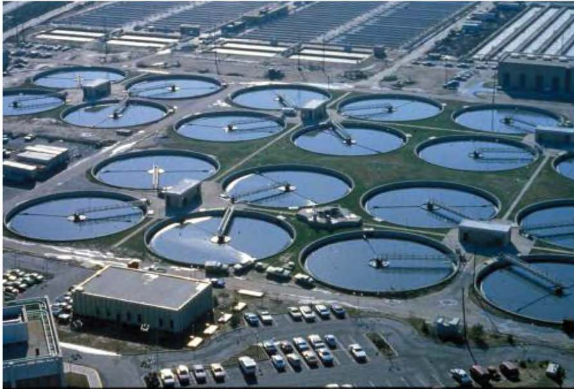
Figure 25.1 Sewage Treatment Plant (credit: "eutrophication&hypoxia"/flickr.com)
