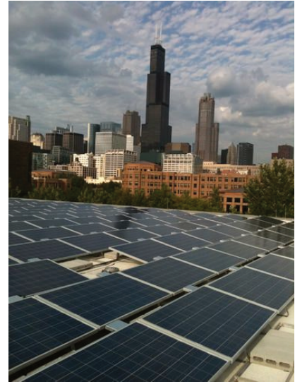
Figure 4. Rooftop Solar Installations Rooftop solar installation on Douglas Hall at the University of Illinois at Chicago has no effect on land resources, while producing electricity with zero emissions. Source: Office of Sustainability, UIC
