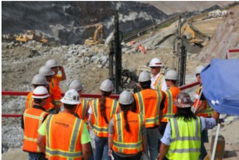
Figure 6.8. Engineering and construction students gather around a job site. How do your academic interests define your in- and out-groups? (Photo courtesy of USACEpublicaffairs/flickr)
