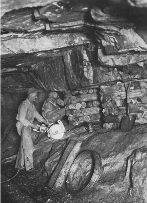
Figure 1. Timber supports in a mine on the Reef, 1920s.
