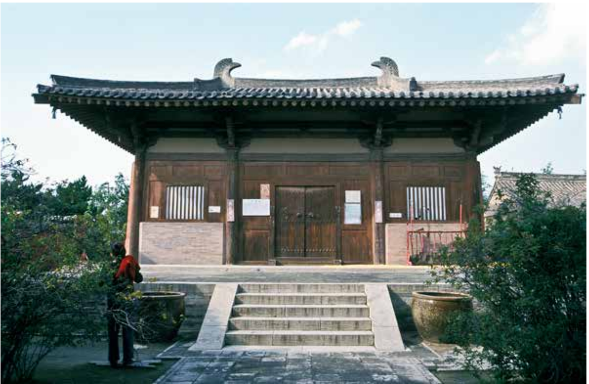
Figure 2.7. Main hall of Nanchansi, 782 C.E., front facade (photo by the author)
