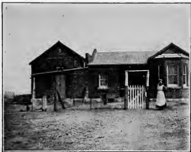
Boxburg Mission Station. Built by Mr. Jesse Eyster.
