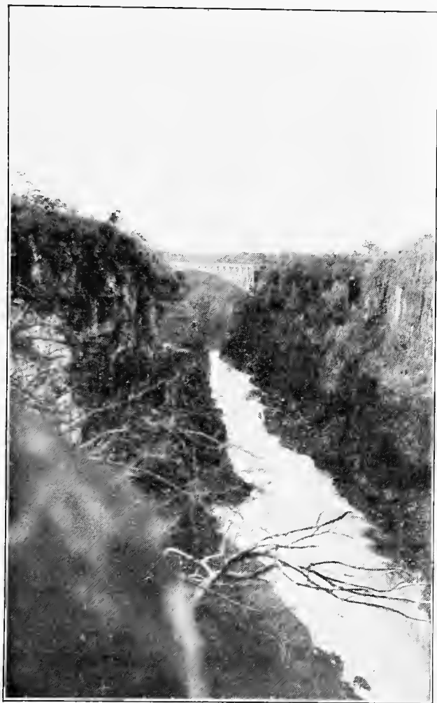
Victoria Falls Bridge.
