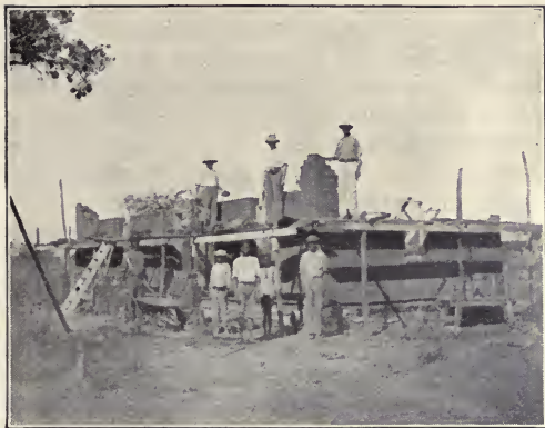
Building the Boys' House at Matopo, M. S.
