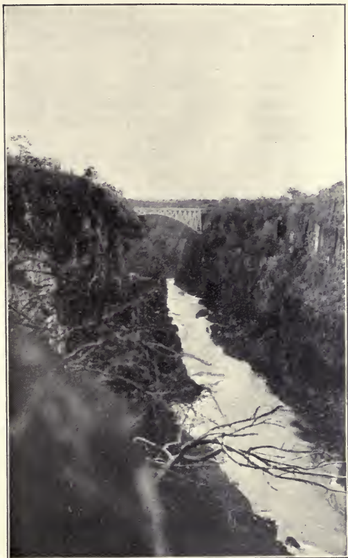
Victoria Falls Bridge.
