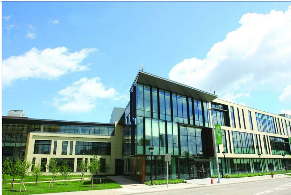
Figure 5.1 Outfitting a New Building
