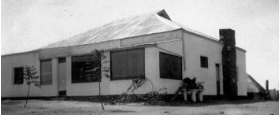
The Sikalongo Mission house as it appeared when the Steckleys began work there in 1925.
