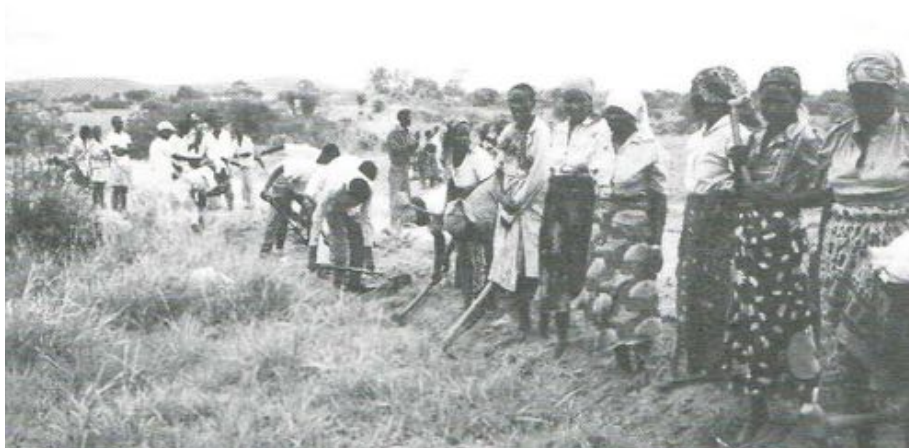
Food for Work road repair project at Sikalongo Mission.
