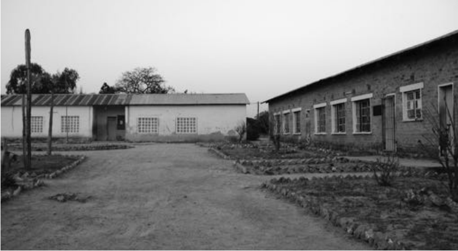
Sikalongo Basic School's old block alongside the new classroom block.
