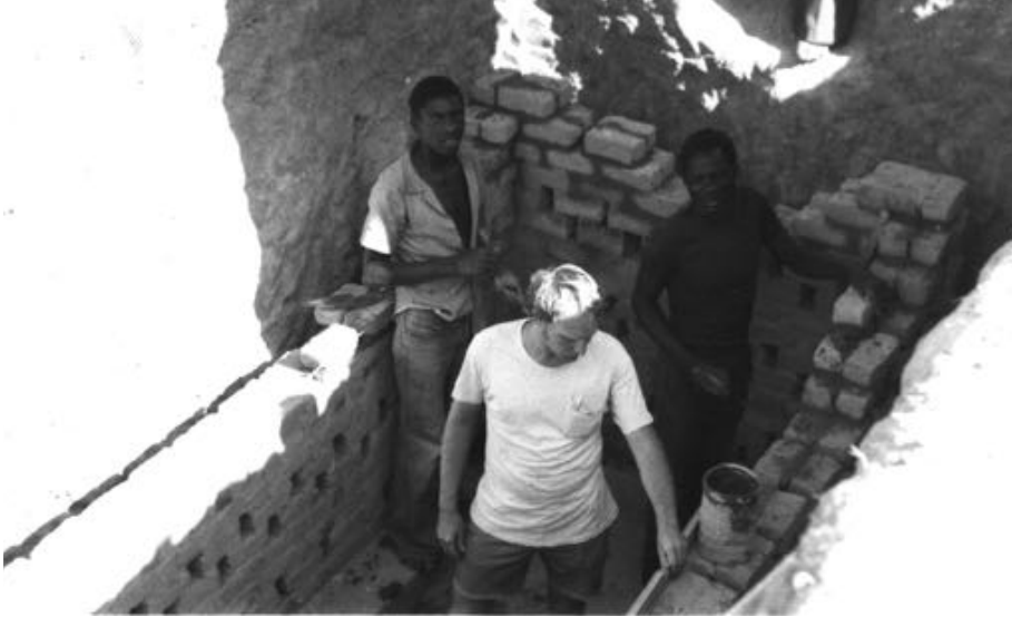
Building the sewage system.
